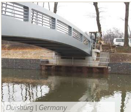
Temporary cofferdam | Germany
